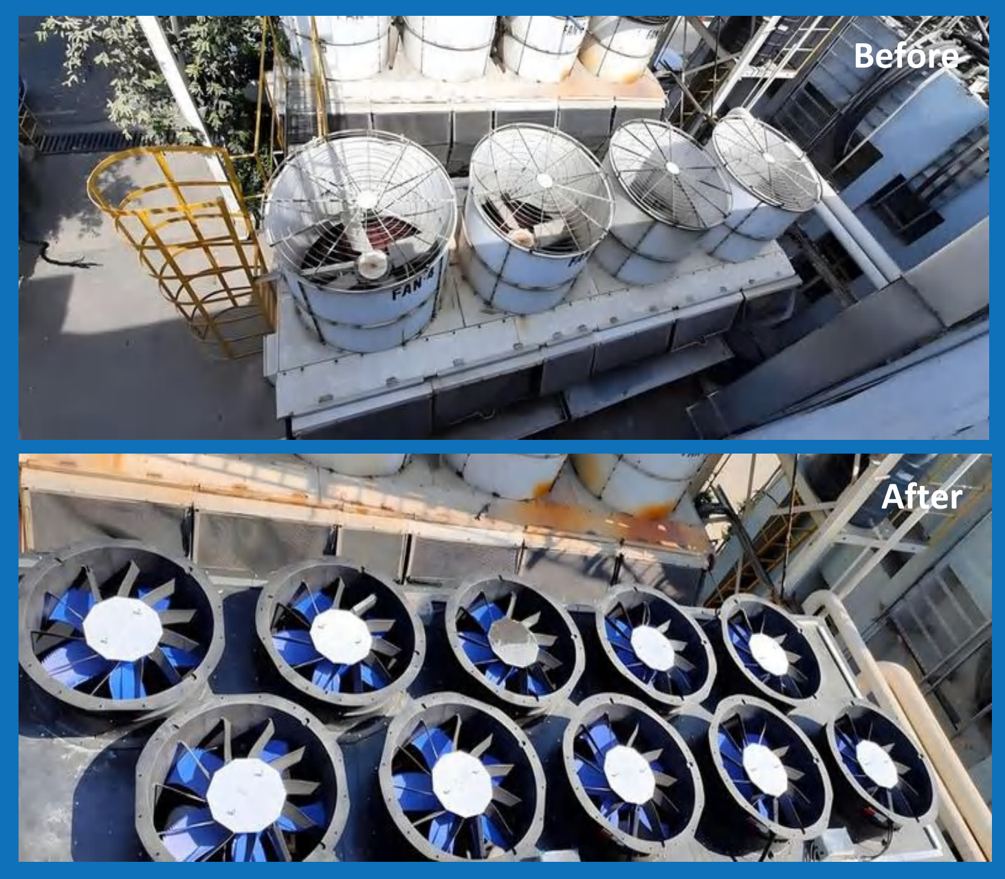
Retrofit Solution in Cooling Tower
