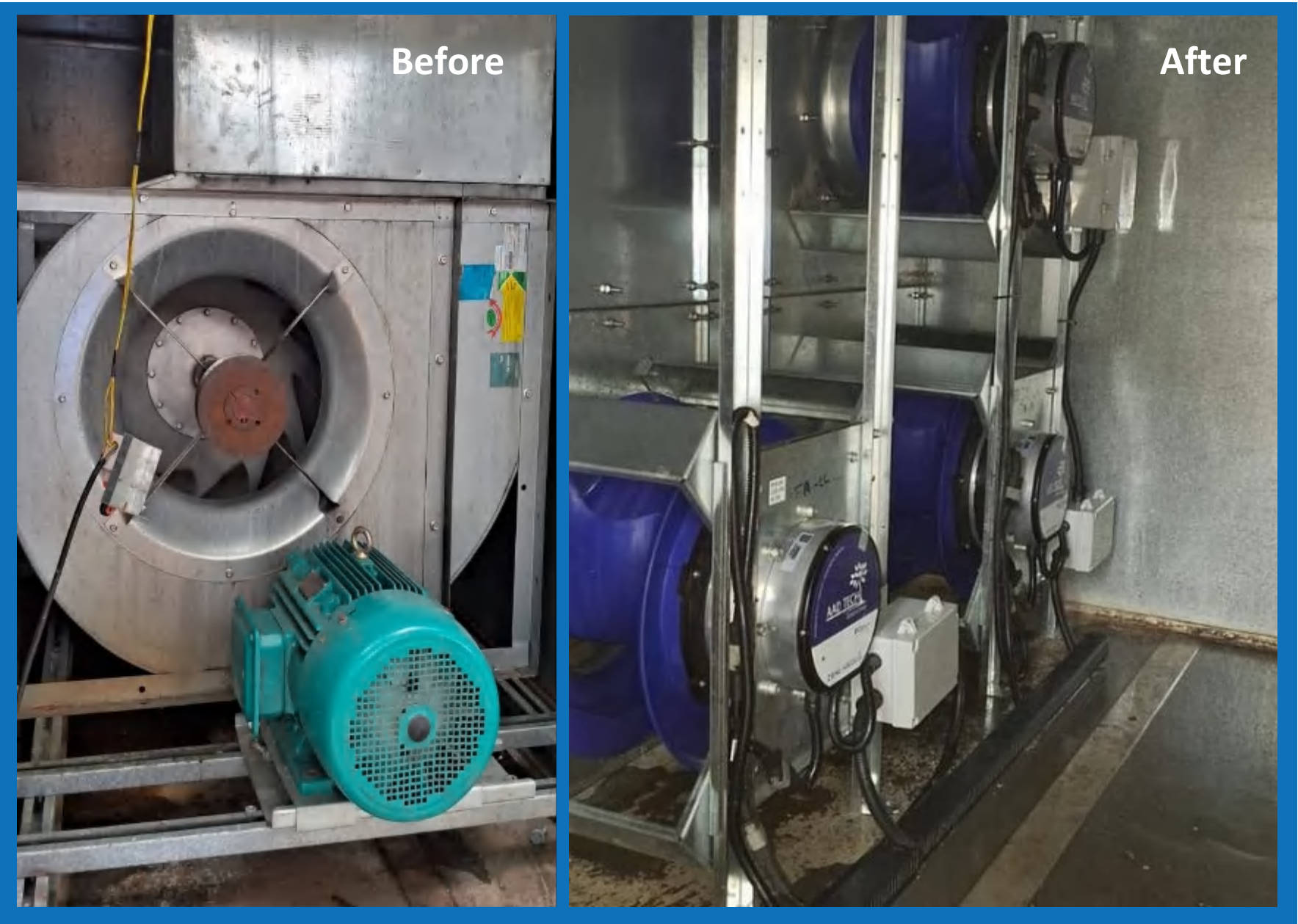
Retrofit Solution in Air Handling Unit
